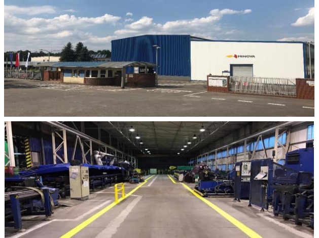
Fig. 1. Manufacturing Plant in Golce.
